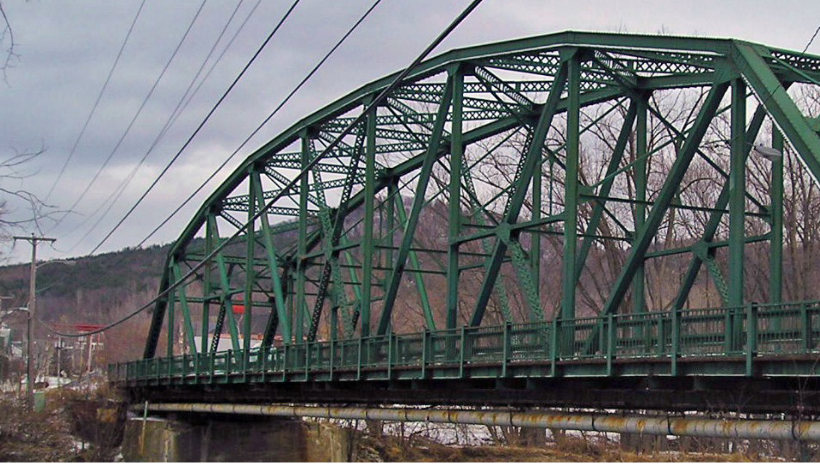
Bridge Street Bridge over Winooski River Rehabilitation, Richmond, Vermont
