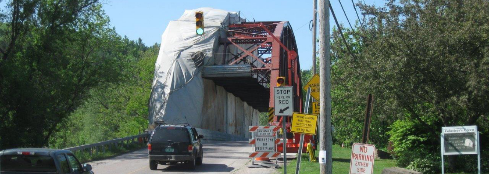
Richmond Bridge Painting, Richmond, Vermont
