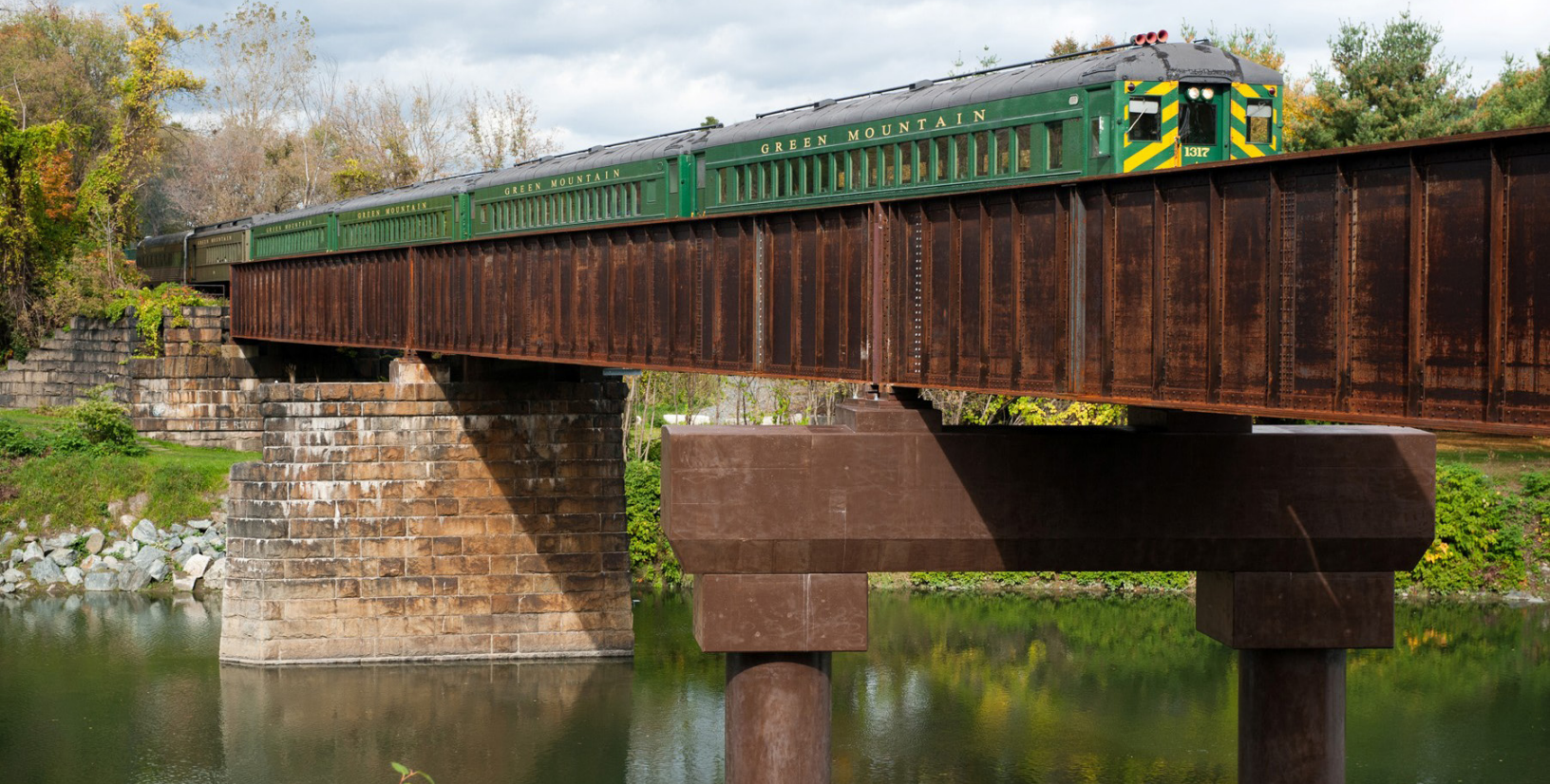
WACR Bridge 501 Emergency Repairs, Hartford, Vermont
